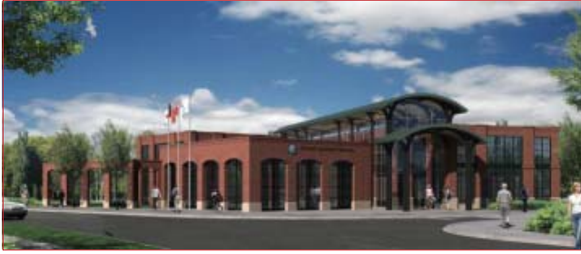
The new Town Hall – loan and grant money helps to get the shovels in the ground
